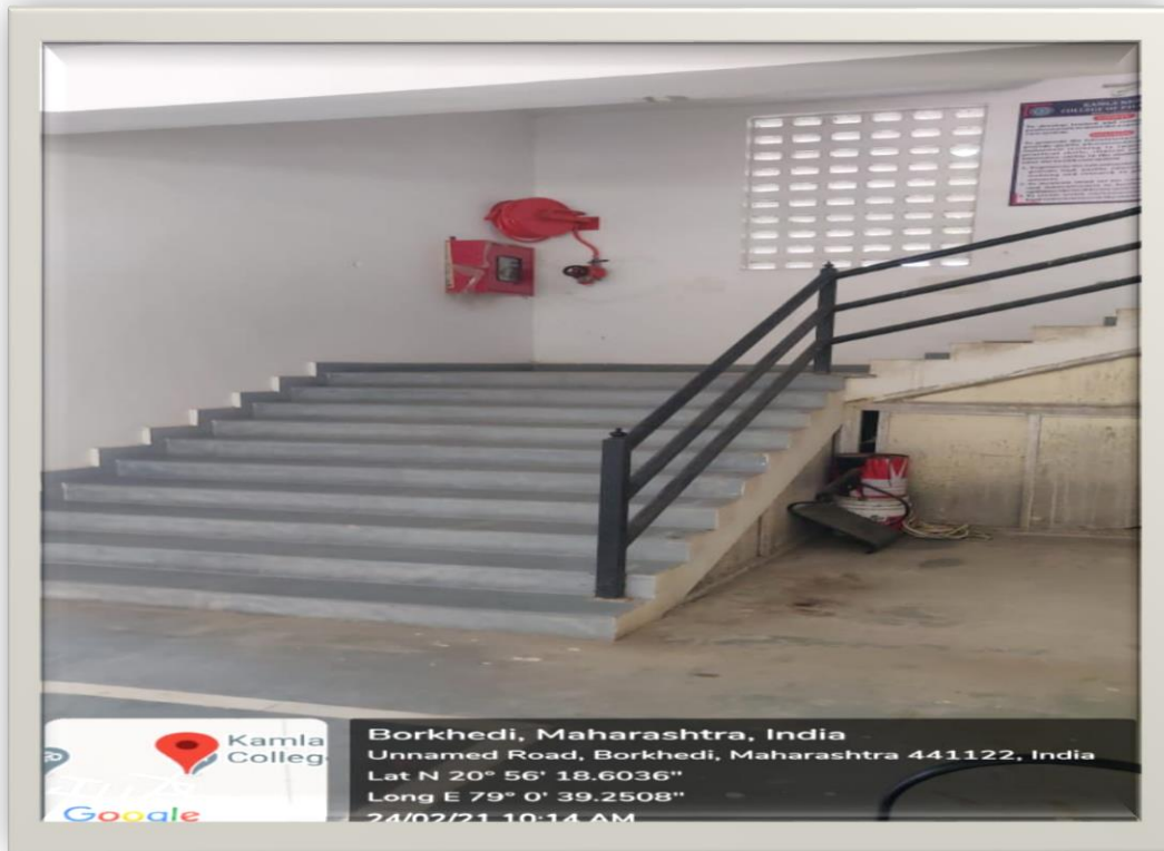
Staircase with railing
