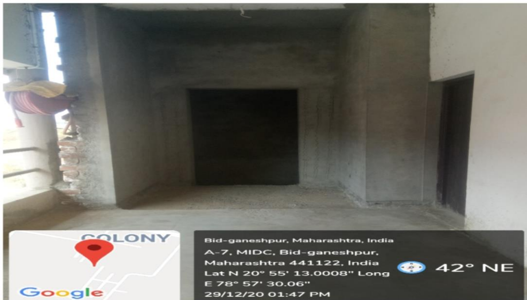
Lift work under progress
